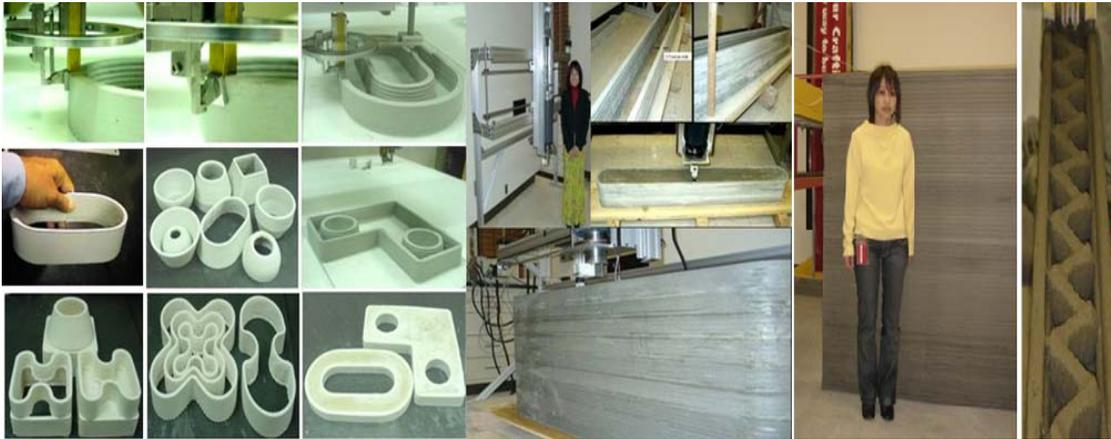
Figure 1 Structures built by Contour Crafting
